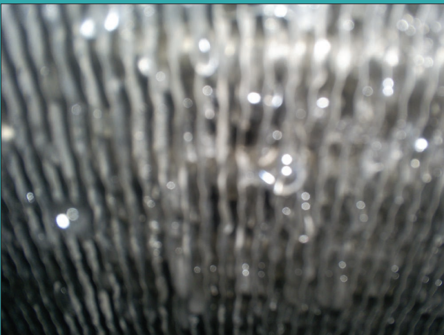
Frost melting from the evaporator coil surface during defrosting.
