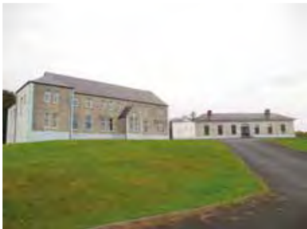
16.2. Coláiste Chonnacht (with the former Arrandale House to the right of picture), Sheeaunroe
